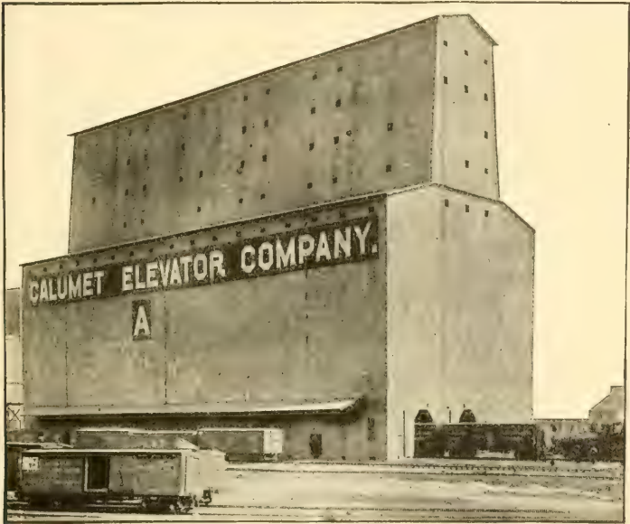
Fig 58—Typical Modern Grain Warehouse
